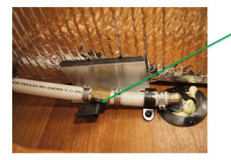
Leave valved closed (as shown in picture) unless you are manually draining your main water tank
