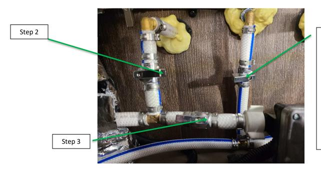
If you have a 2<sup>nd</sup> water tank, turn this value to the open position to manually drain the 2<sup>nd</sup> water tank.
