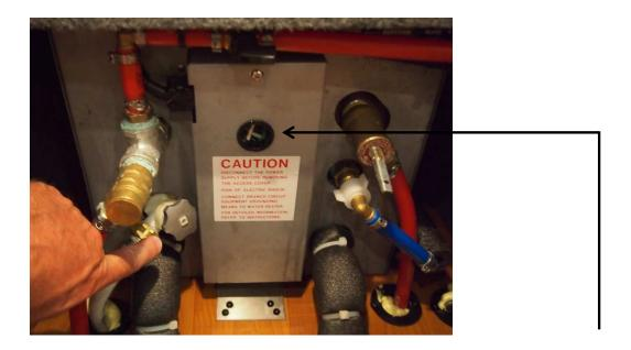
Try to remember not to engage the lighted water heater switch while the engine block is still hot; by doing this, you take the risk of tripping the reset breaker on the thermostat of the water heater. The <u>reset button</u> is located on the water heater unit, accessible through the small hole on the front panel of the water heater shown in the above picture.
